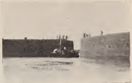
Locks in the Grand Canal, Tsing-kiang-pu, China. House boat being pulled by wire cable worked by man power.
